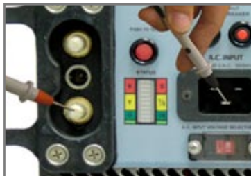
3.8.7 - Negative Probe on the AC Ground Post and the Positive Probe on the DC Positive Post.
