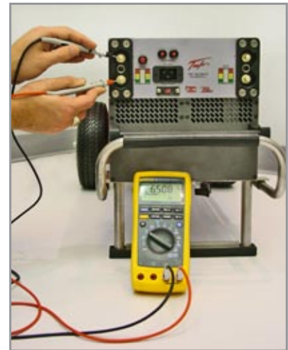
Figure 3.8.2 – Testing DC Receptacle
