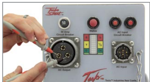
Figure 3.7.6: Testing DC Voltage Reading
