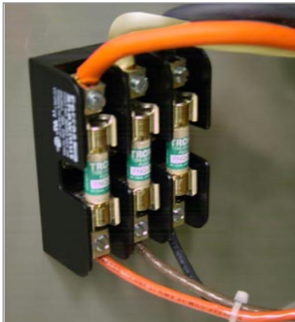
Figure 4.4.1 Replaceable Fuses
